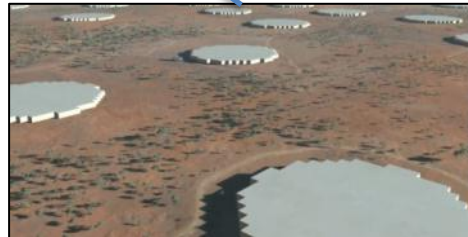
SKA2_AA 250 x Mid Frequency Aperture Array Stations
